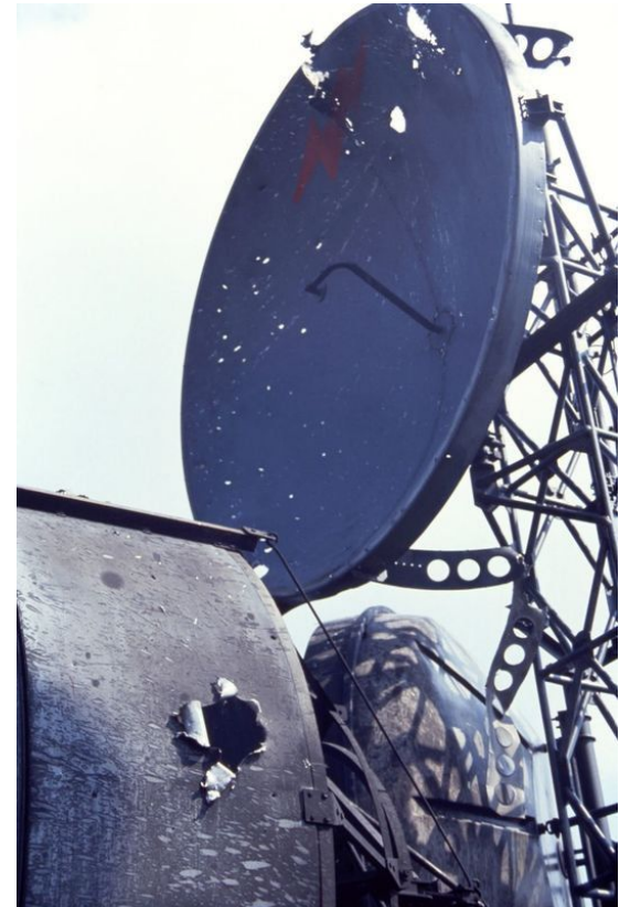
Communication station “Kum” damaged by JNA air raid on 2 July 1991
